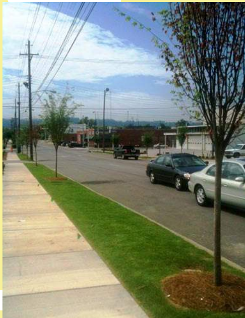
A new 14th Street emerges during construction.
